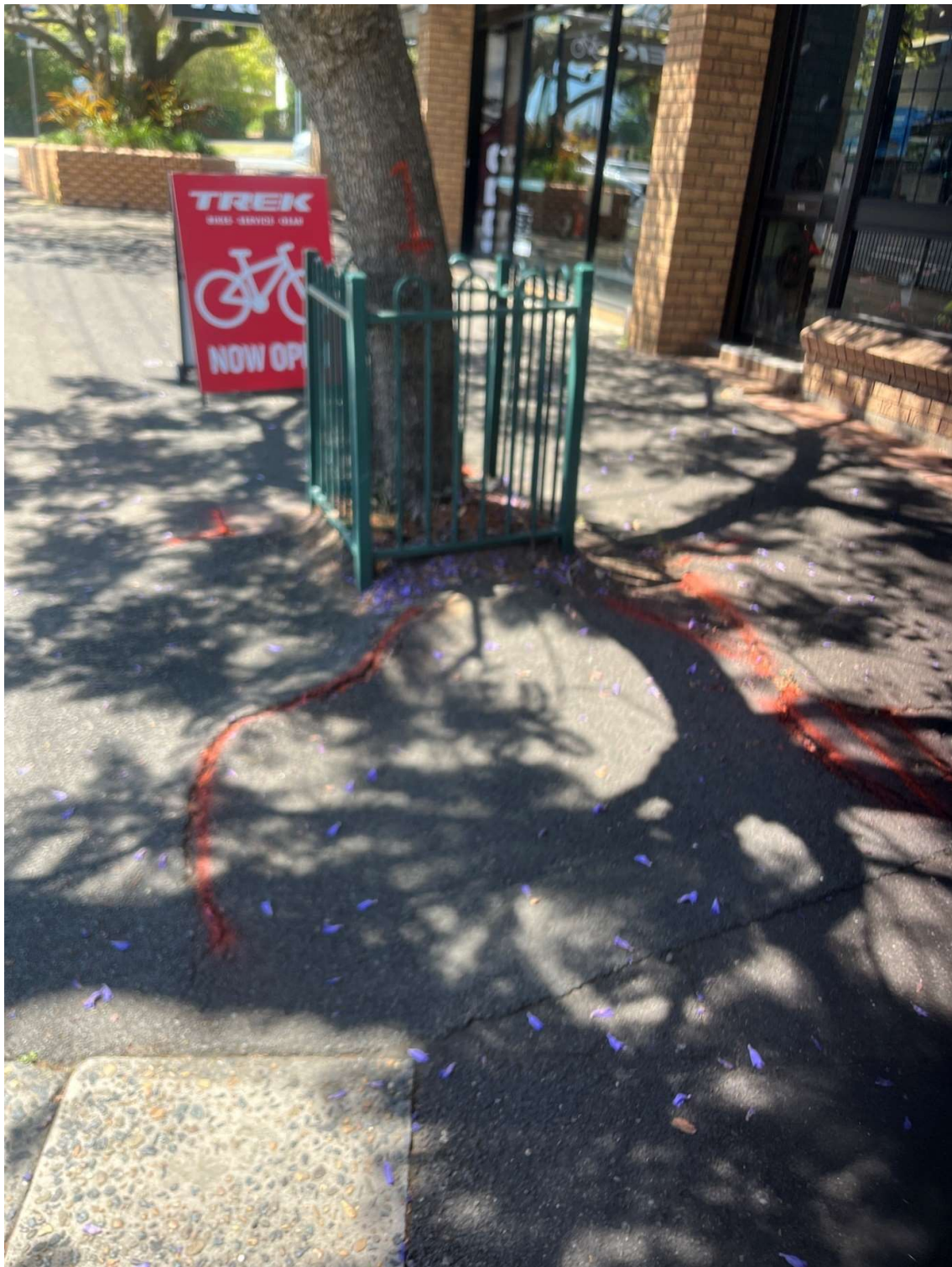
Tree 1 – Jacaranda mimosifolia - Lifted pathways due to root impact.
